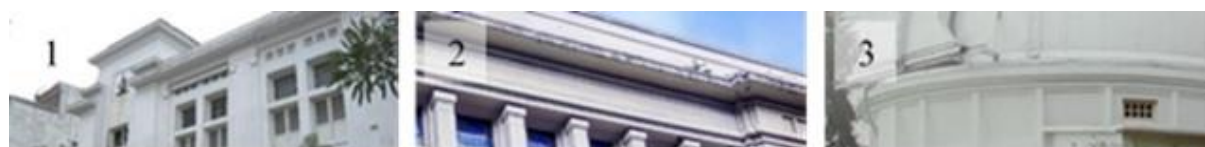
Gambar 21. Becker & Co. Building (1), Van Dorp Office Bookshop and Print Shop (2), Bosscha Observatory (3)
