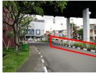
Gambar 20. Material Beton (Concrete) (sumber : hasil survey, 2017)
