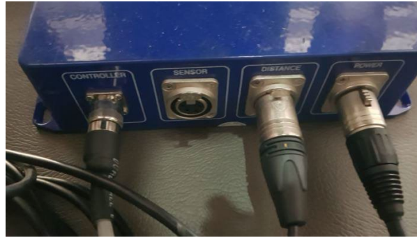
Fig. 6. Power Cable Installation
