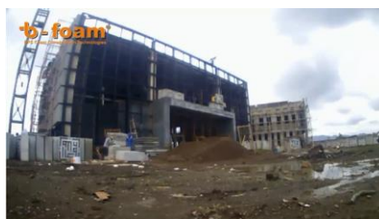
Gambar 18 Proses pemasangan Frame Sumber : https://www.youtube.com/watch?v=XpWsv_cbiMM
