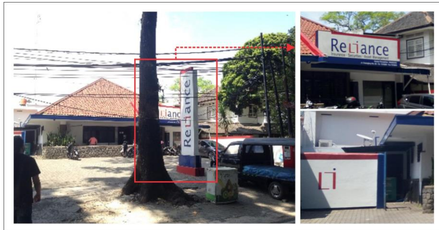
Gambar 10. Bangunan C3 (Reliance)
