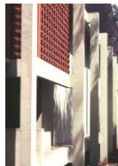
Gambar 4.12 Material Beton Krawang
