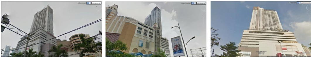
Gambar. 2 : Tampak apartemen Cosmo Terrace (Sumber : survey 17 november 2015)
