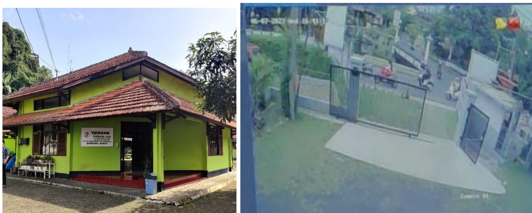
Figure 1. Some parts of the school require CCTV installation
