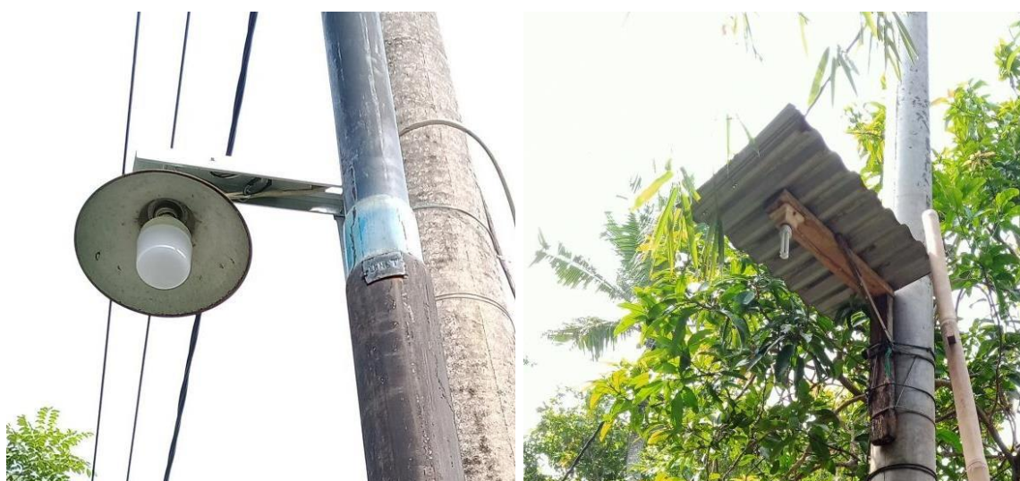
Figure 4. Process and Results of Installing
