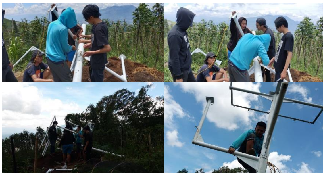
Figure 5. Solar Power Tree construction installation process
