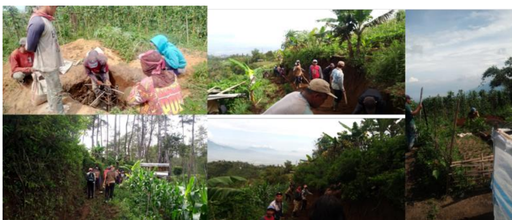
Figure 4. Road widening process and making Solar Power Tree foundation
