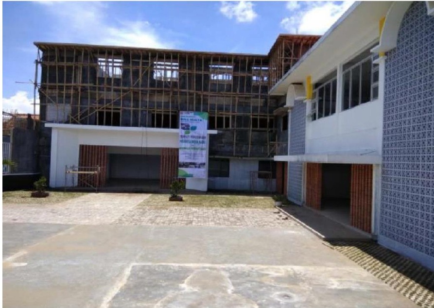
Figure 1. The process of building the YBTMA Boarding School.
