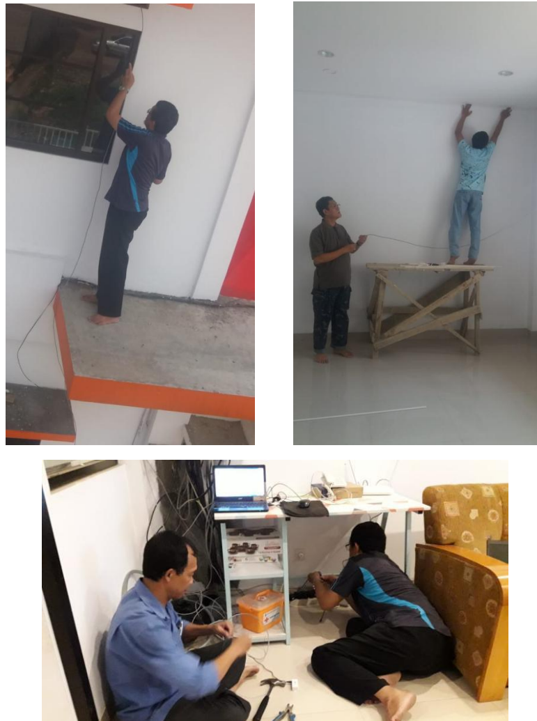
Figure 2. Installation of hotspot and access points
