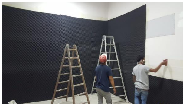
Figure 4. Foam Installation for Soundproof
