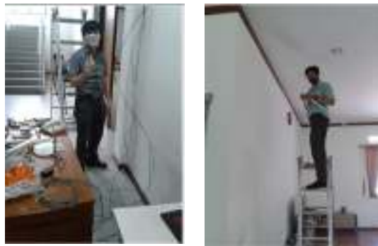
Figure 6. Installation of Fibre Optic and Telephone Cables on The First Floor and Installation Access Point on The Second Floor.
