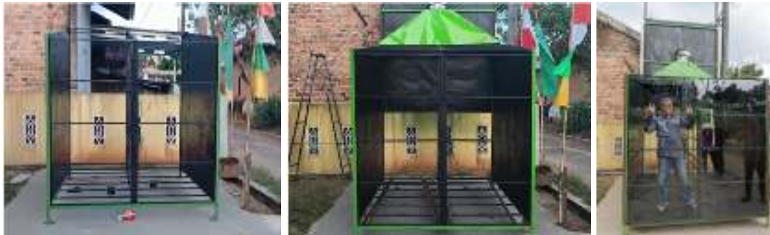
Figure 8. Wall, Ventilator, Glass and Floor Installation
