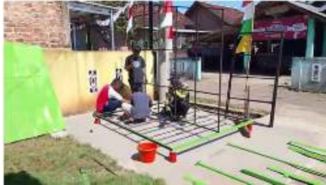
Figure 7. The Process of Assembling the Base Frame and Legs
