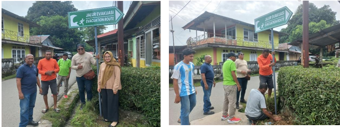
Figure 5. The service team together with the community are installing evacuation direction signs.
