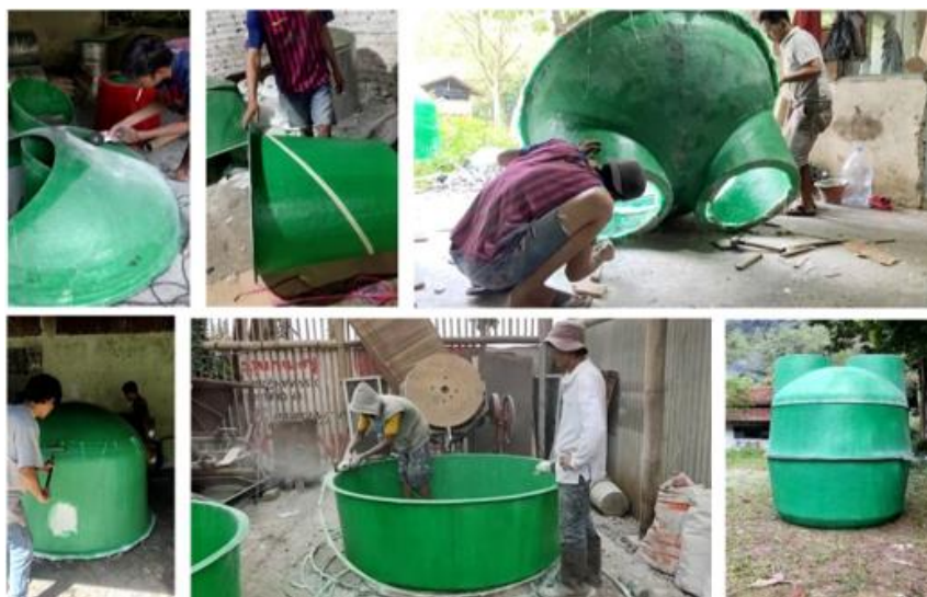
Figure 3. Manufacture of FRP biogas reactor
