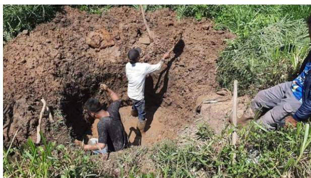
Figure 4. Excavation of holes for reactor installation
