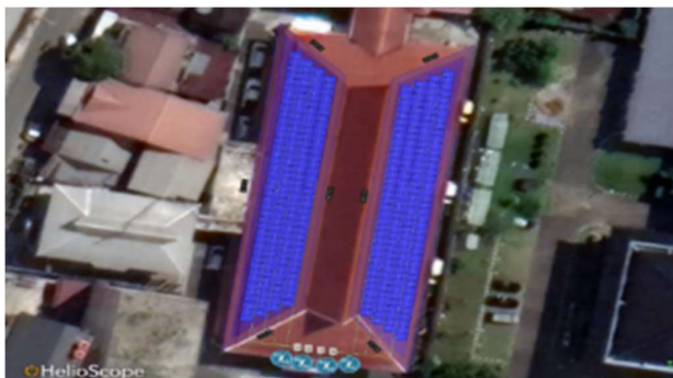
Figure 6. On-Grid Rooftop Solar Power Plant System on Office Building of PT. PLN (Persero) UP3 Samarinda
