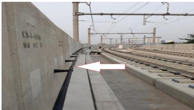
Gambar 1. Leaky Coaxial Cable (LCX)
