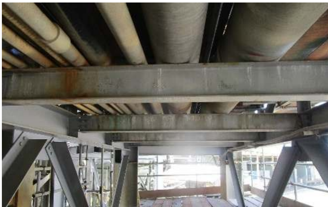
Gambar 2. Strudur baja piperack .
